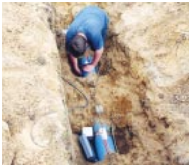
WORKING WITH ANGLIAN WATER - UEA HELPS SOLVE UNDERGROUND PIPE PROBLEMS
